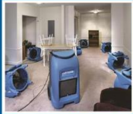
Structural Drying
